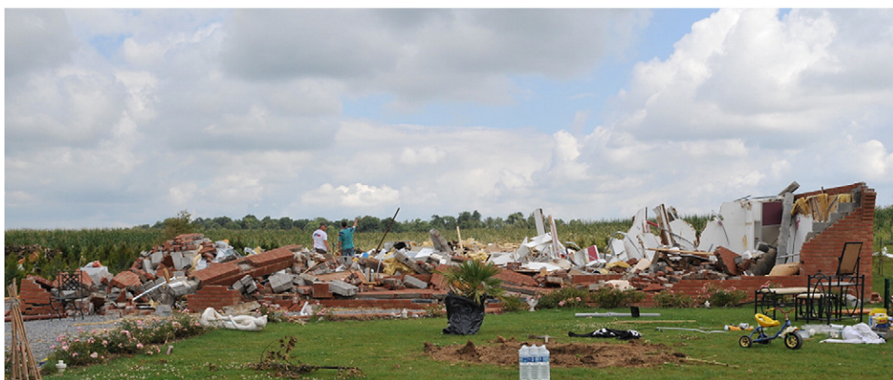
Fig. 1. Total destruction of a solidly built house in Boussières-sur-Sambre (F4 intensity).
